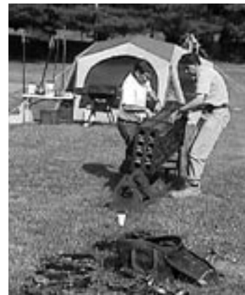
Joe Tracey, KB3LNM and Norm Lorenzen KB3KZG prepare to raise a tower. The cage holds all the tubes, and fits in the base section for storage. Photo by W3YRS.
